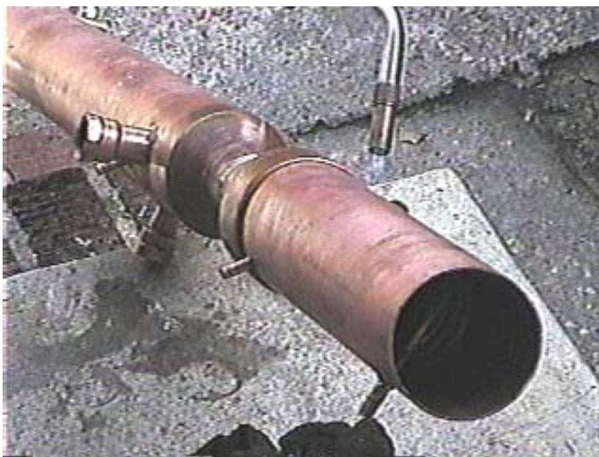
This is the condenser section being soldered into place, after gently tapping it inside the 3-inch midsection joint. Read on further, as it doesn't get attached yet.
